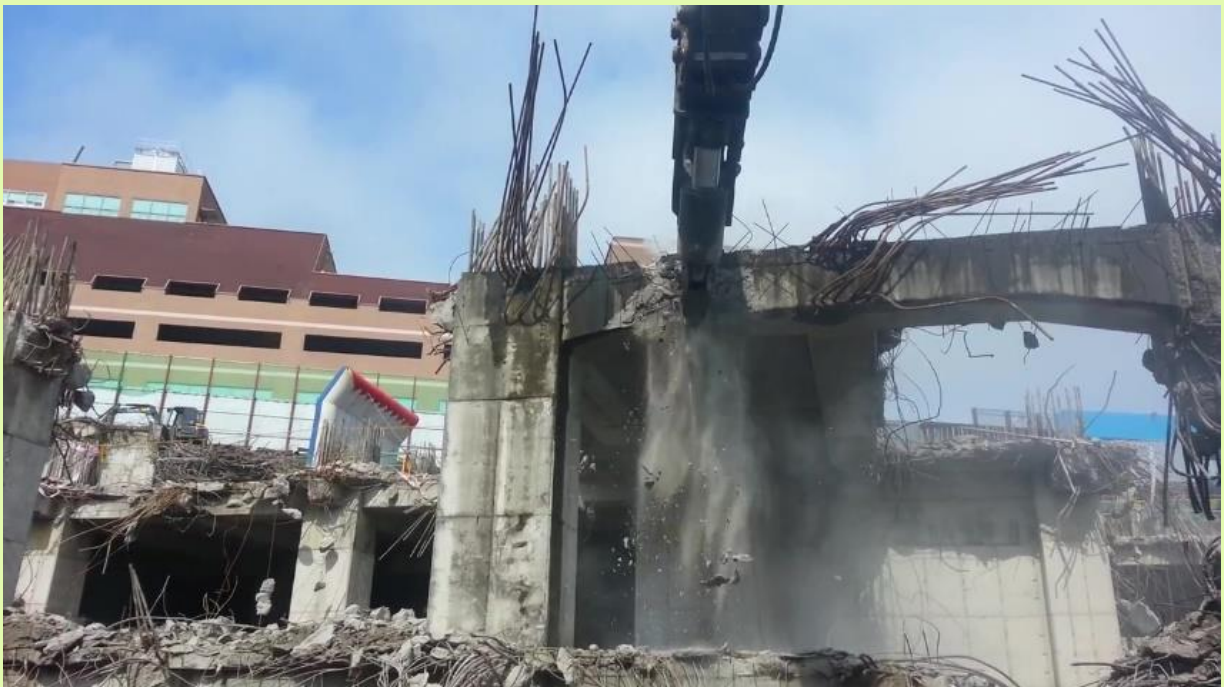
Demolition of the huge reinforced concrete structure of the Parking lot
