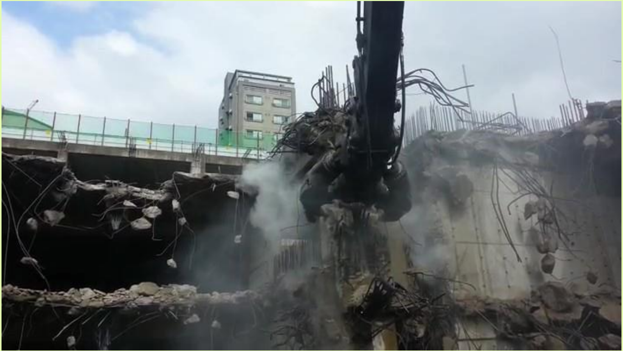
Demolition of the huge reinforced concrete structure of the shopping mall
